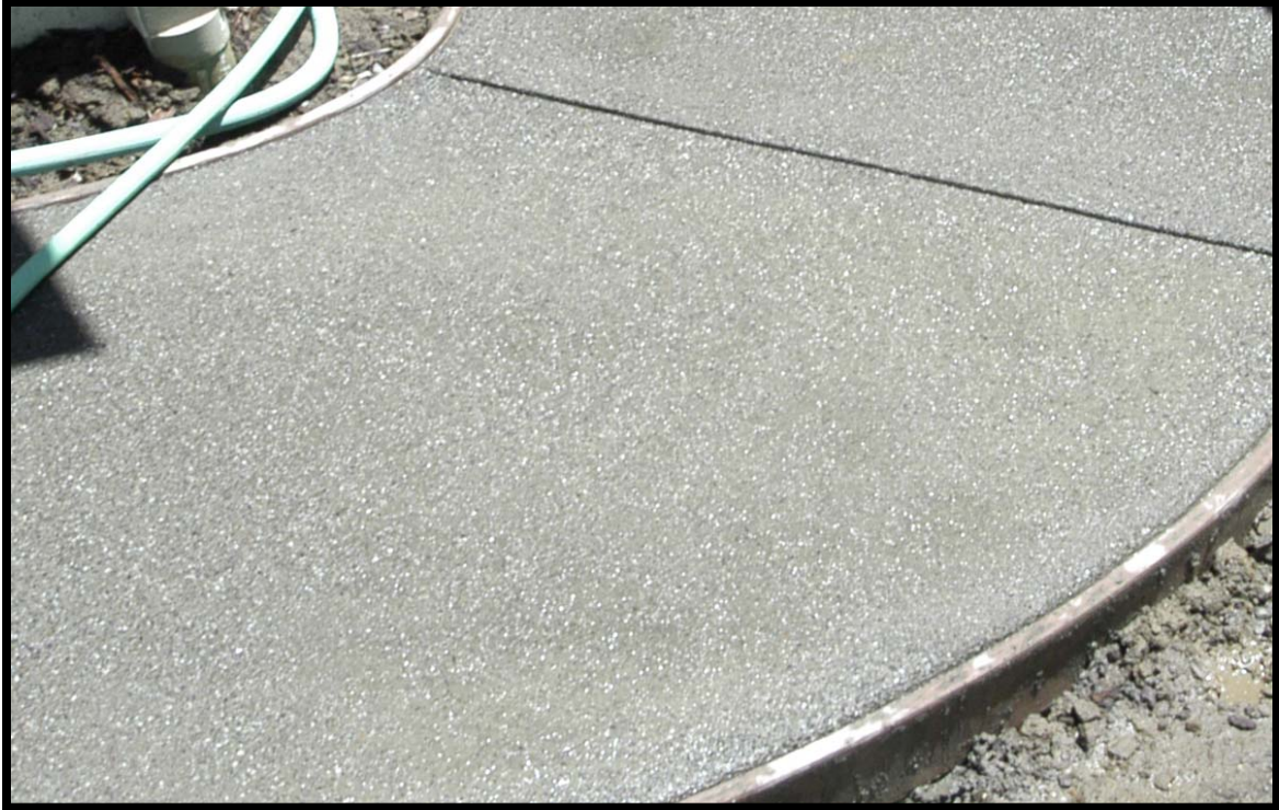
Exposed Aggregate Concrete Finish
