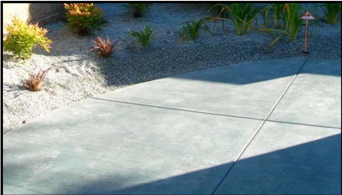
Dust on Colored Concrete with Broom Finish
